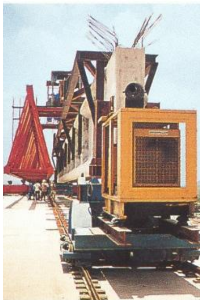
Figure 2. Placing of bridge structure using railway.
