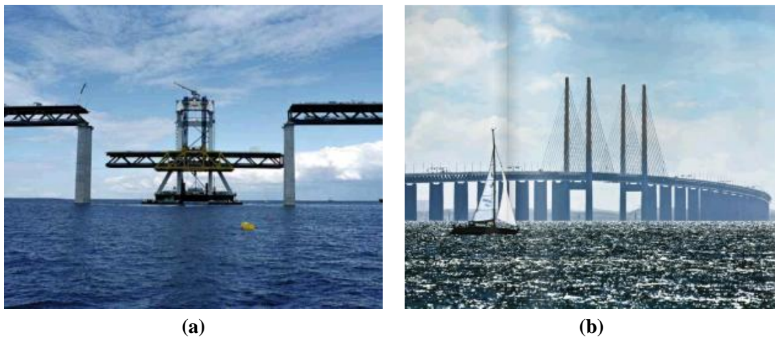
Figure 4. Öresund bridge (Sweden – Denmark): (a) photograph of ship which is carrying bridge structure during its construction; (b) photograph of final bridge in service.
