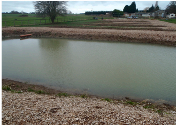
Figure 2. The finished excavated swales in preparation for planting, 2013.
