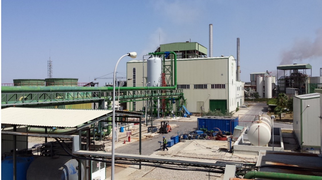
4 5 Figure 1. View of the incorporation of HCT at the “Vetejar” biomass power plant.
