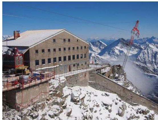
Figure 2.5. Refugio de Torino, Italy [13]
