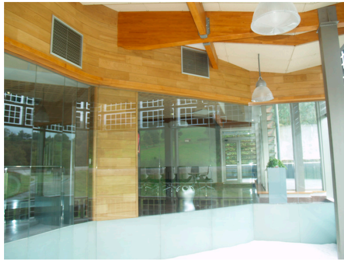
Figure 3. Interior wall (partially glazed) in the attached sunspace.
