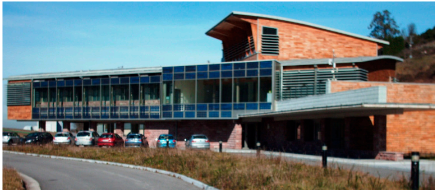
Figure 1. Demonstration container with attached sunspace (south side) located at San Pedro de Anes, Asturias (northern Spain).
