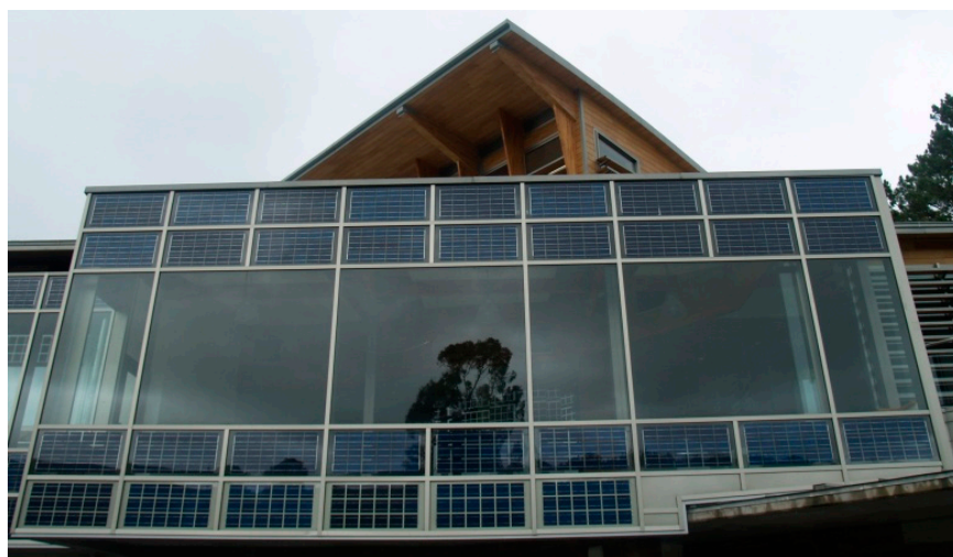
Figure 2. External glazed surface of the attached sunspace in the demonstration-container.
