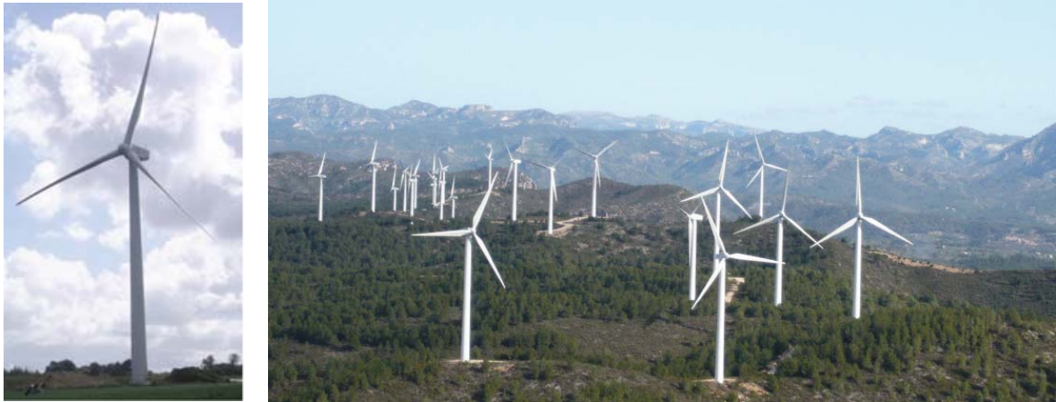
Fig. 1. General view of the Abuela de Santa Ana wind farm and one of the towers
