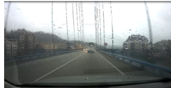
(b) Image of the road on a rainy morning
