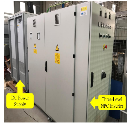
Fig. 8: Test bench for overmodulation strategies: a) Schematic representation of the laboratory setup; b) 4 kV/40A three-level NPC ELINSA inverter.
