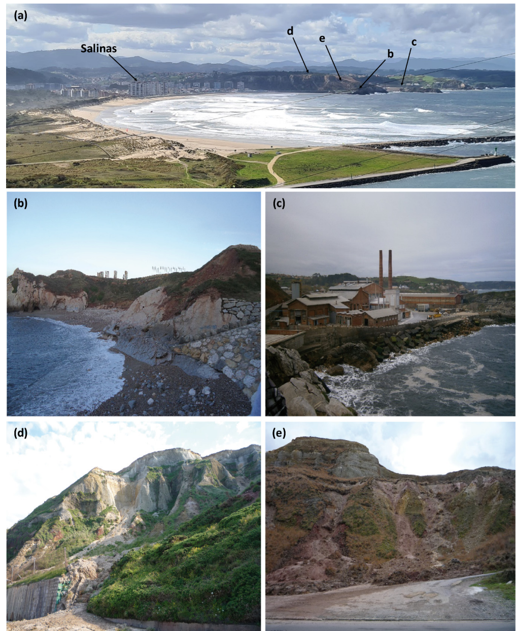
Figure 6. Salinas area views. (a) Salinas town panorama; (b) cliffs and beach of La Peñona; (c) industries located at the El Cuerno beach; (d) and (e) debris flows on the Salinas-La Peñona road in 2010 and 2008, respectively.
