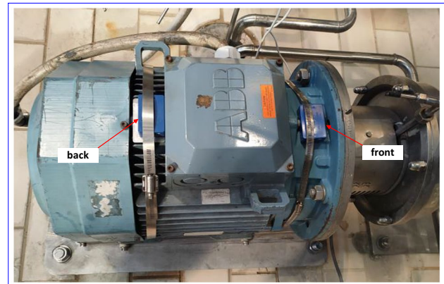
Fig. 5 Scenario 2: multi-sensor modules locations
