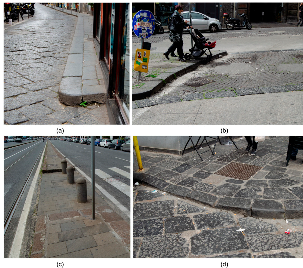
Figure 2. Architectural barriers in the metropolitan city of Naples: (a) narrow pavements, (b) kerbs, (c) obstacles at zebra crossings, (d) uneven level crossings.
