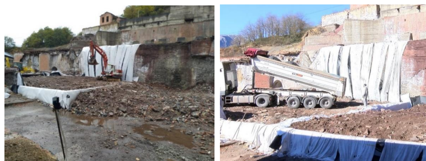
Figure 12. (Left): task 6 (excavator in rubble), (Right): tasks 7, 8 (dump truck).
