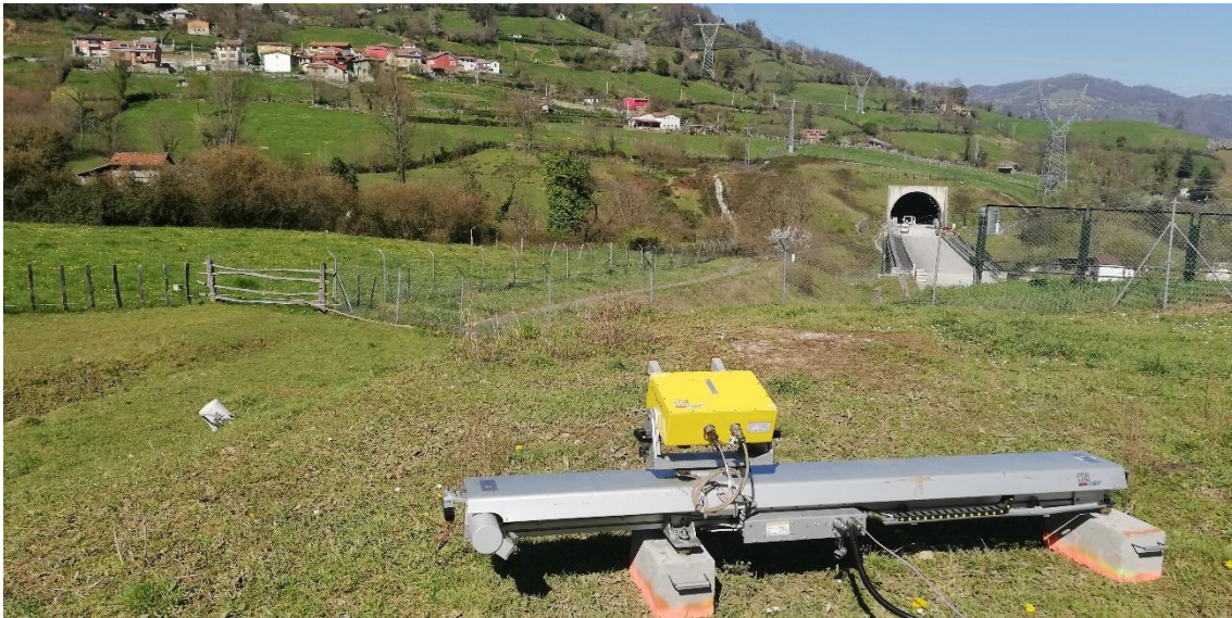
Figure 50. Ground-Based SAR used to detect slope instabilities in Mamorana (Aller, Asturias). SEDTRIGE Project (Ref. FUI-19-128) carried out by GEA Asesoría Geológica S. COOP. ASTUR and co-funded by IDEPA (Ref. IDE/2018/00385).
